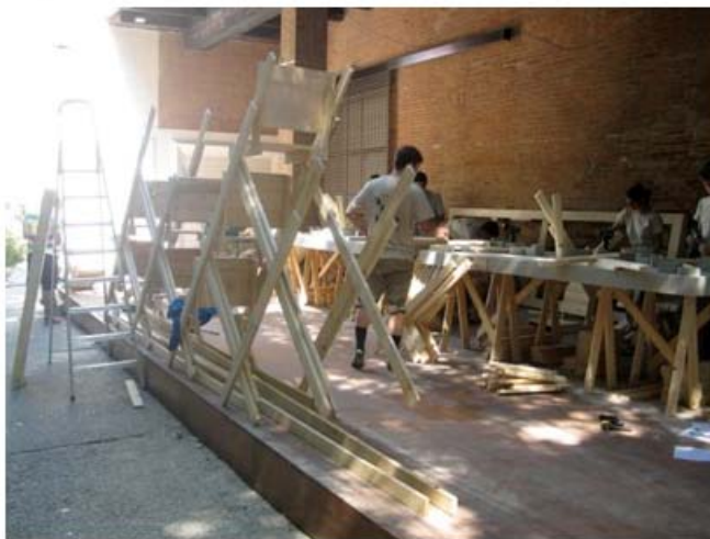
Stair-chairs under construction by the Raum Berlin crew.
