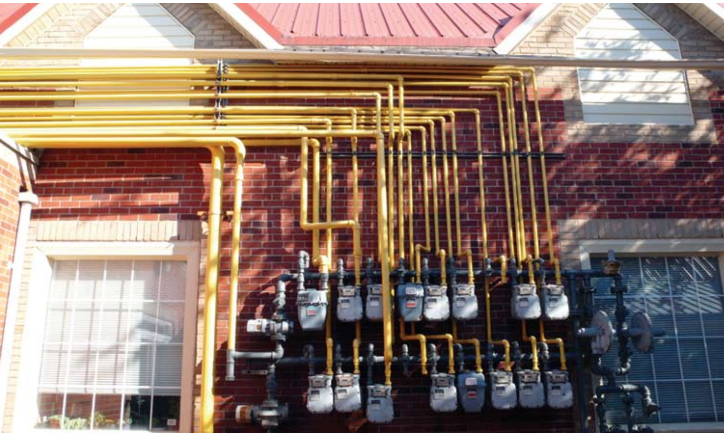
13 Each yellow-painted gas line represents one restaurant or food kiosk inside the vast and sprawling Pacific Mall in Markham, a successful mall that caters to Markham's largely Asian community
