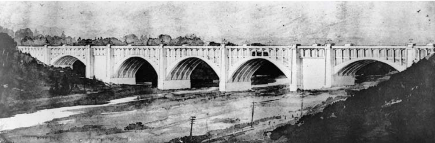
22 John M. Lyle's reinforced concrete bridge proposal for the Bloor Viaduct (c.1911)
