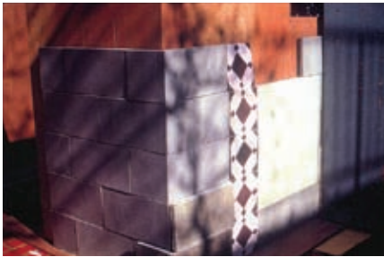
8: Construction mock-up of a building corner, showing concrete, plaster and tile. HNA, 1989.
