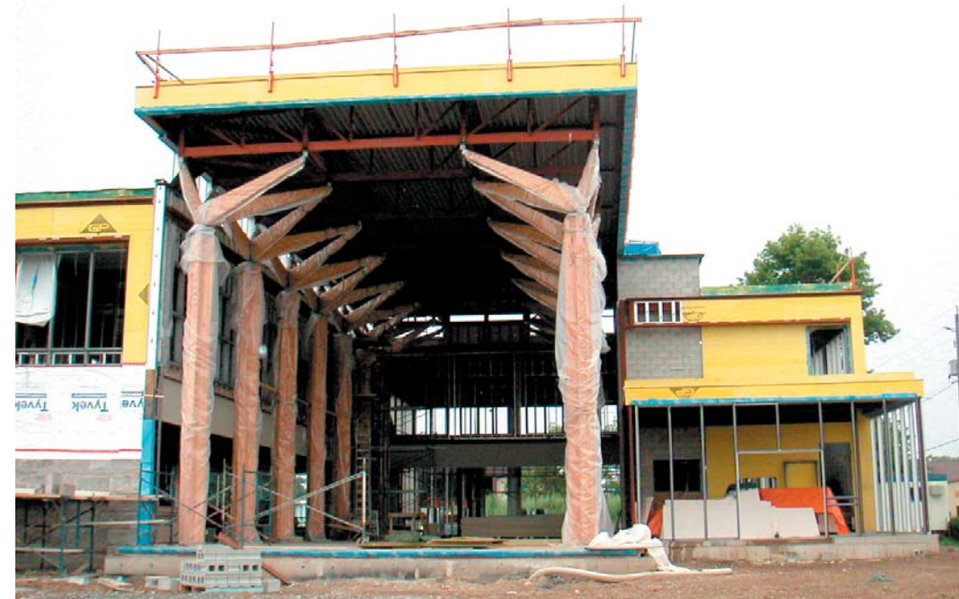
Figure 2 Construction phase; glue-laminated columns framing into roof structure
