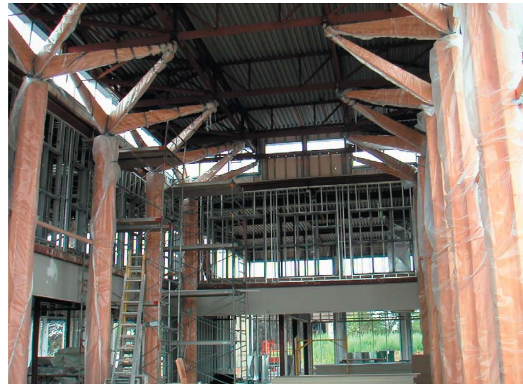
Figure 3 Detail, installation of columns
