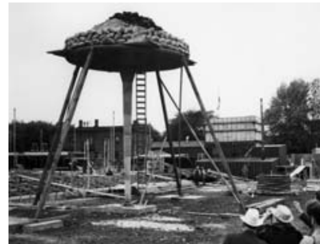
Fig. 1.4 Frank Lloyd Wright witnessing the load testing a prototype concrete column for the Johnson Wax Administration Building
